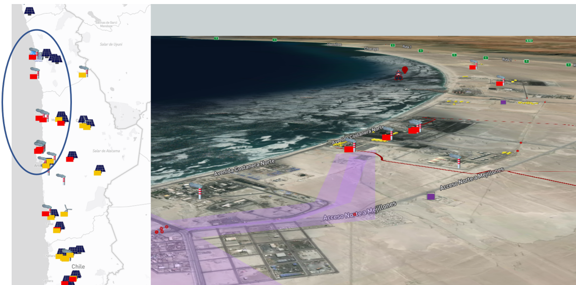
Figure 8: Size and location of thermal power plants in the north of Chile.
